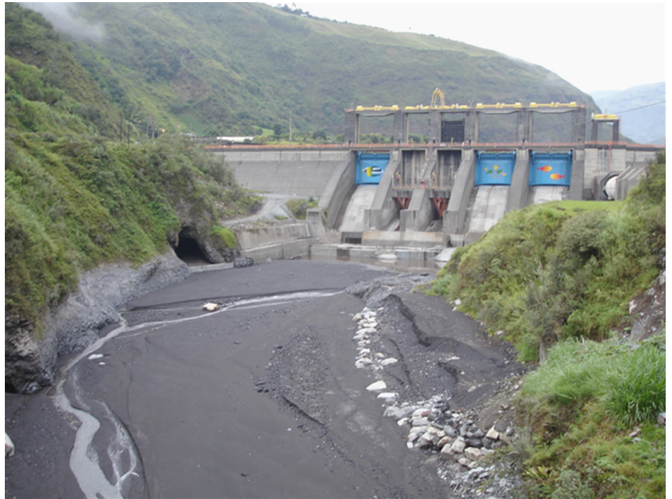
Fig. 1. Hydropower Dam in upper Amazon Basin, Ecuador © 2009 Elizabeth Anderson.
